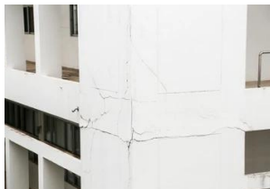
• Structural cracks
