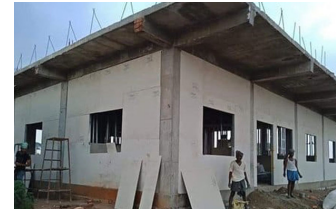
• Cement Board joints
