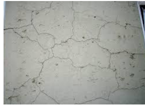
• Plaster cracks
